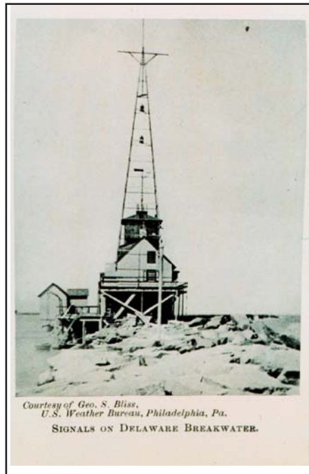
Picture 1 - Signal Tower for Storm Warning Flags used by day, lanterns by night. Used to warn mariners in: "The Boy and the U.S. Weather Men", 1917, p.236. Photo Courtesy of U.S. Weather Bureau circa 1910.
